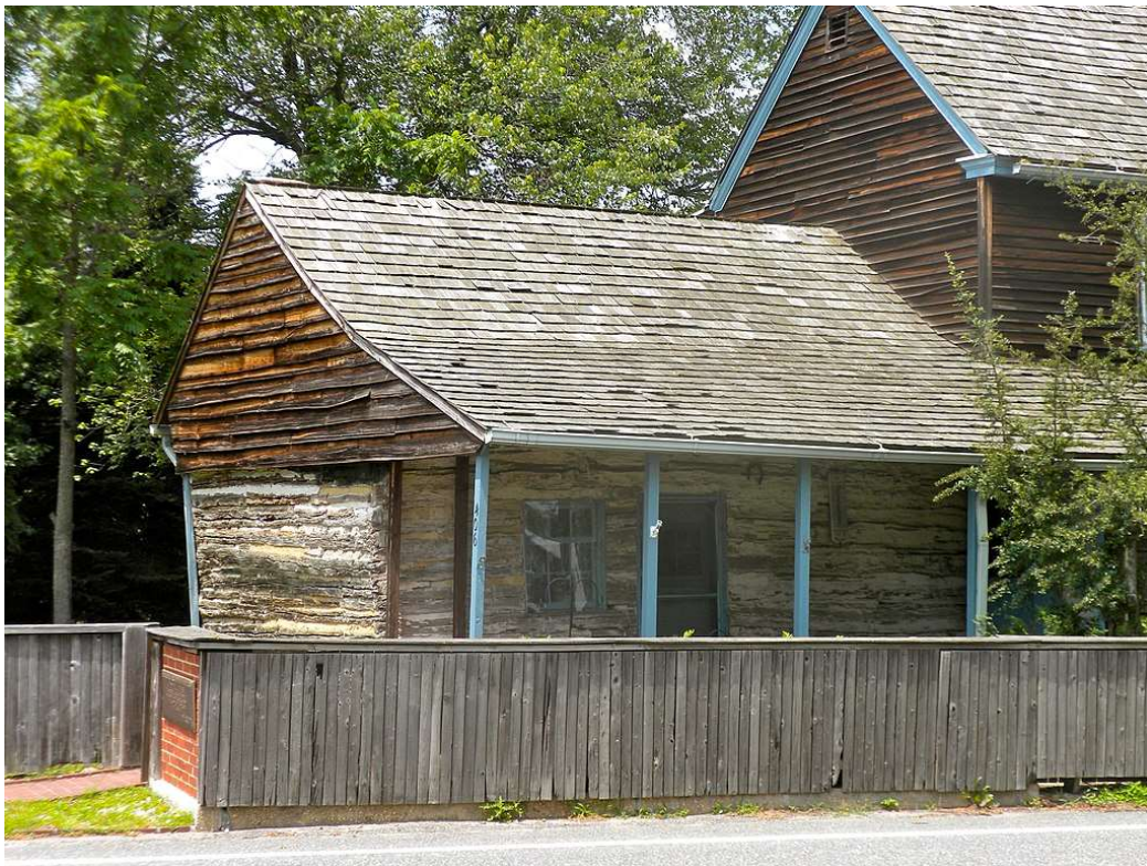
C.A. Nothnagle Log House, built 1640 near Swedesboro, NJ. Oldest surviving log cabin in America.
